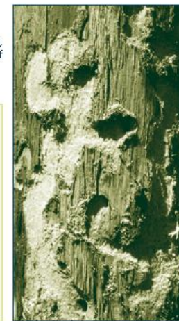
Damage under the bark. Photo: C. Monier
